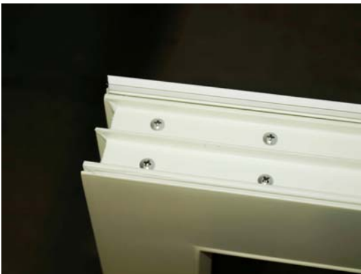
Step 1- Tap the coupling strip into the groove
